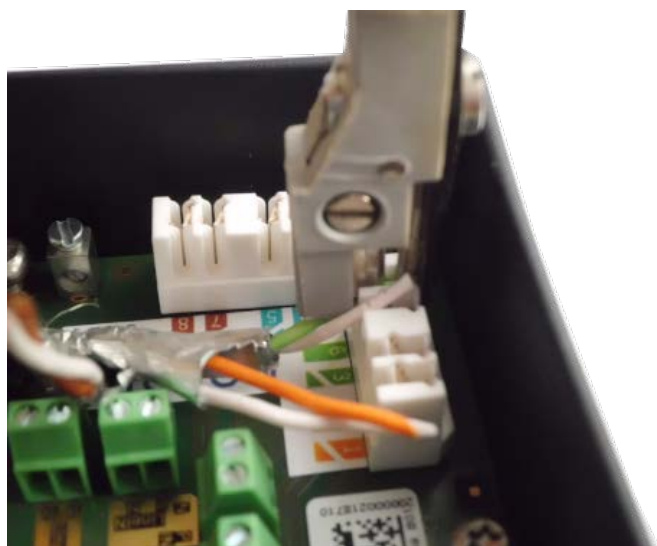
Fig. 26: Network wires connected using LSA+/Krone tool
