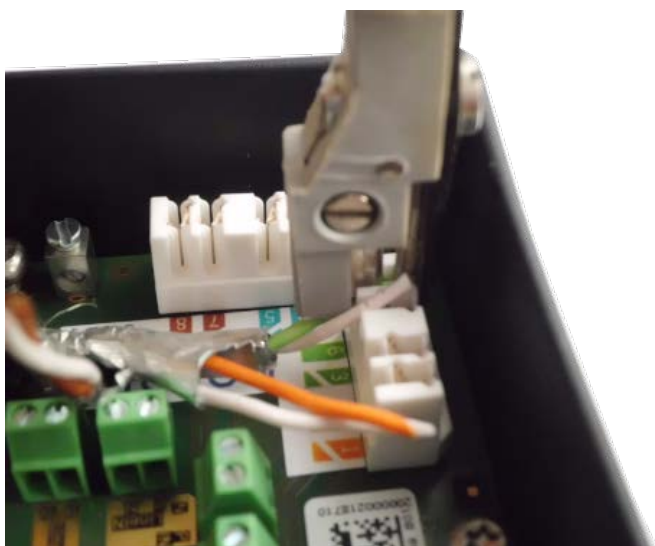
Fig. 26: Network wires connected using LSA+/Krone tool
