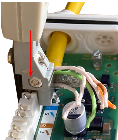
Fig. 13: Network wires connected using LSA+/Krone tool
